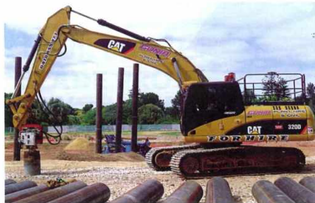
Piling works to support future structures
